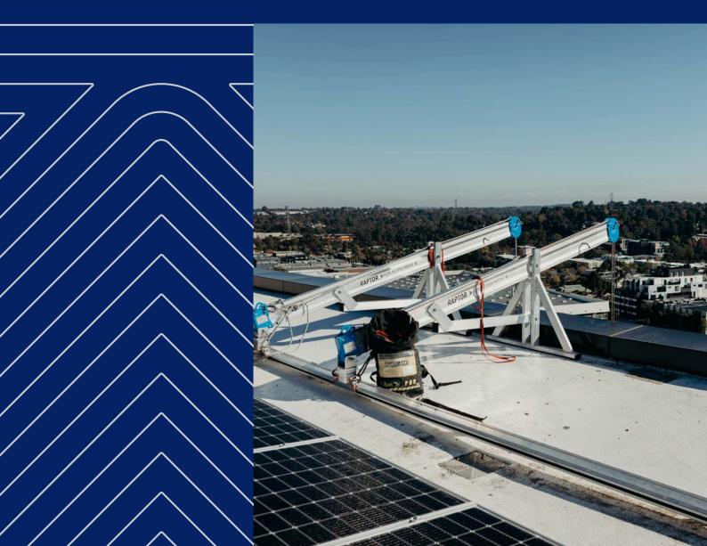
Kattsafe needles are a mobile rope access system providing safe access to building facades in multiple configurations.
