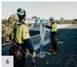
Mounting options Designed to work with many different davit bases including floor, wall and cast in options.
