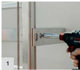
1 Front and rear t-slot attachment on stile
